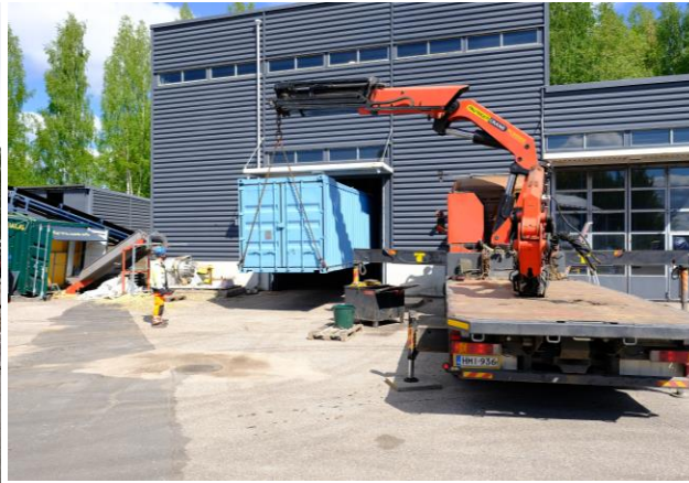
The kiln container was moved to correct position with two cranes (another crane is in the building)
