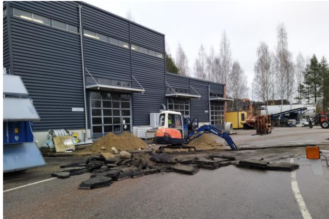
Excavation work for cabling and water
